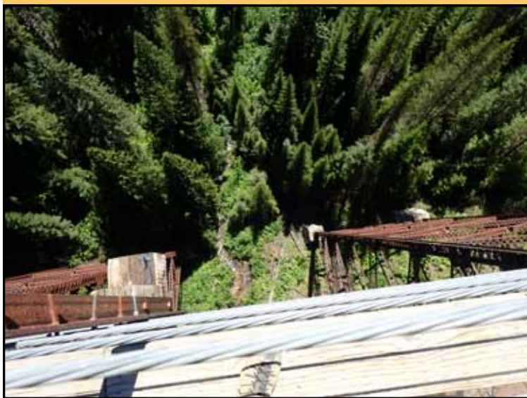
Looking down from atop one of the 7 trestles we would cross. Photo by Roger Crandall
