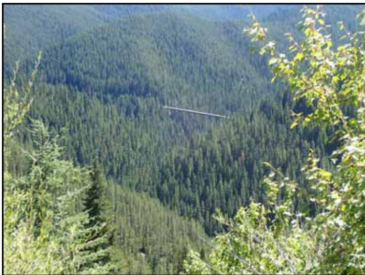
Steel trestles that are for bikes only. Photo by Roger Crandall
